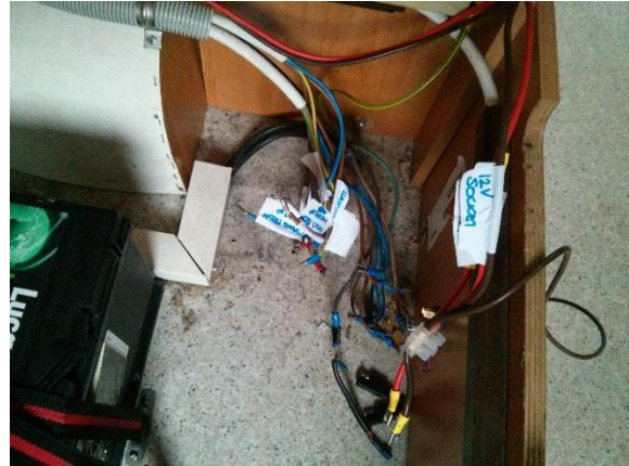
BIP unit removed and cables labelled
